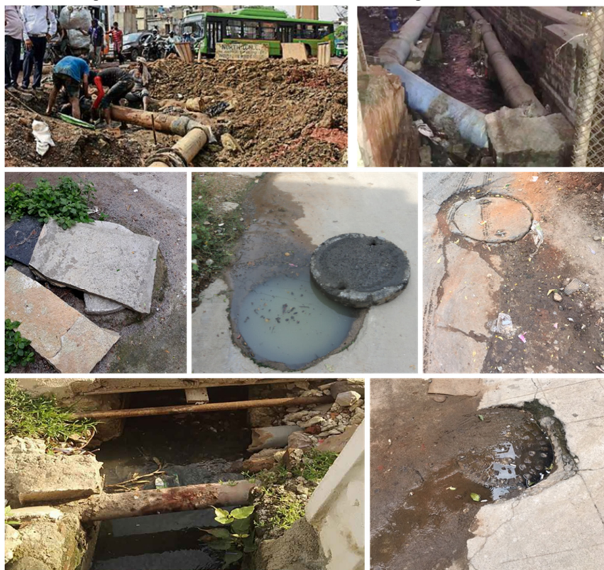
Figure 2: Choked street-sewers & damaged water lines
